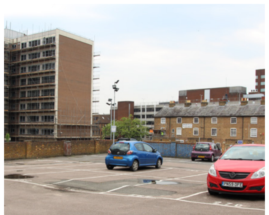
From centre of site looking north-west towards Romney Place
